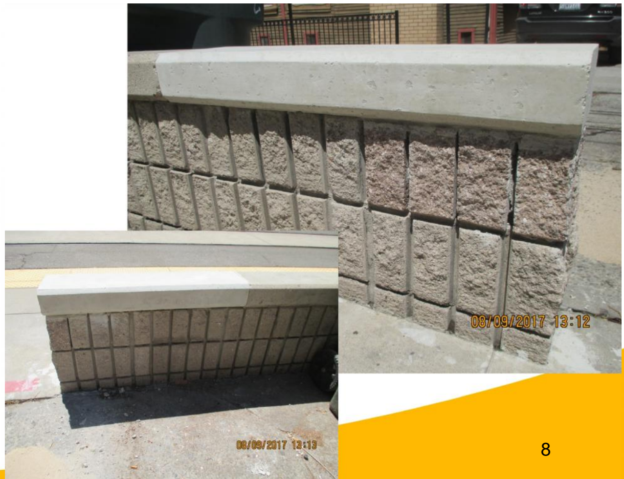
After: Replaced blocks and cap
